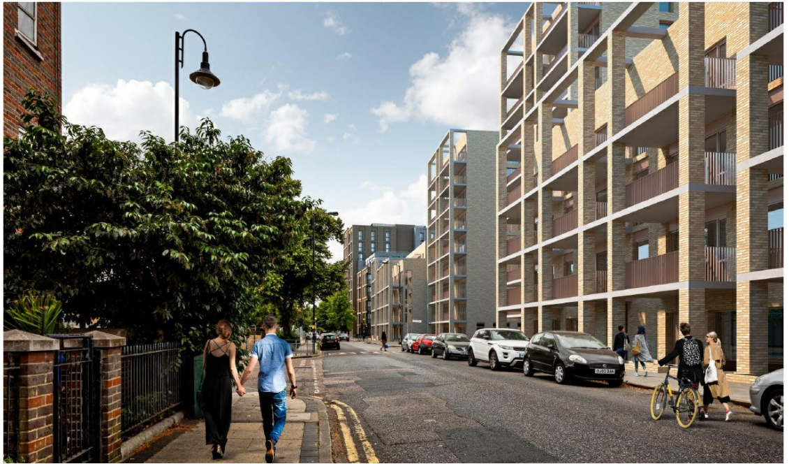
View from Commercial Way outside the approved and under construction 16/AP/4207 site looking east towards the application site. (Note: render reflects massing at initial submission)
